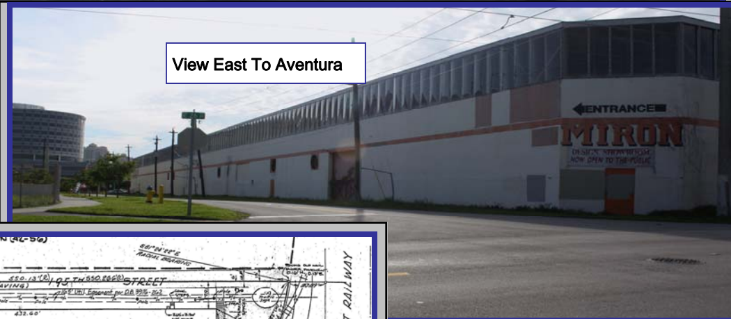
Partial Warehouse View
